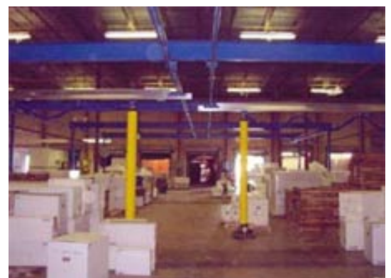
Distribution centre. Palletising with side by side freestanding cranes.
